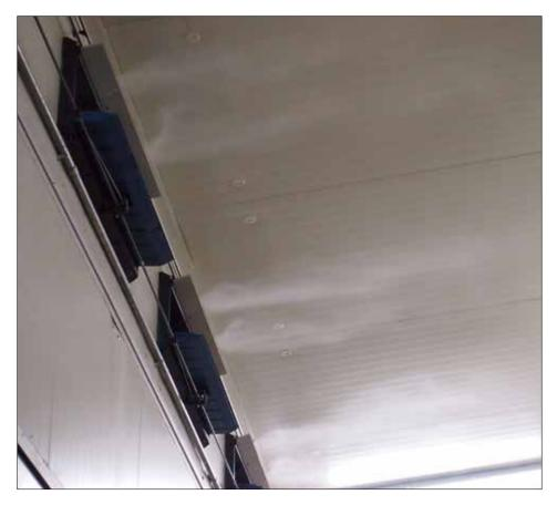
The high-pressure nozzles are installed on pipes in the Rack & Pinion opening and in this way an efficient cooling is created that is easy to regulate.
