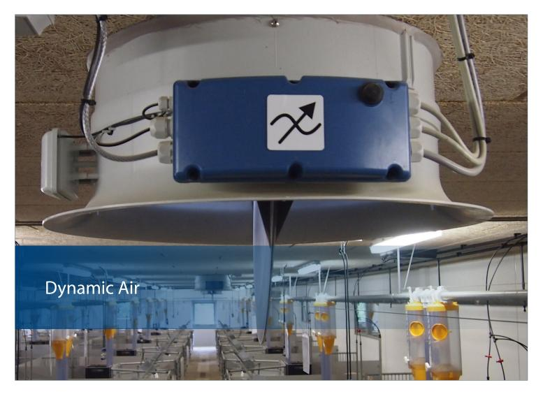
ynamic Air is a measuring method that ensures a correct minimum ventilation for pig producers as well as optimal heat consumption by using precise and constant measurements of air output in the exhaust unit.
