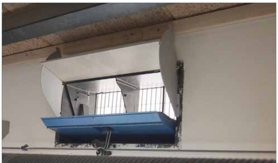
The SKOV air inlets may be used for all kinds of pig production and contribute to ensuring an optimal climate in the livestock house.
