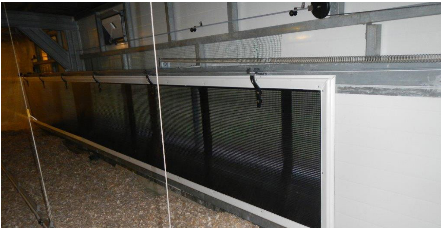
Tunnel Door Light is SKOV's lightweight system for tunnel openings.
