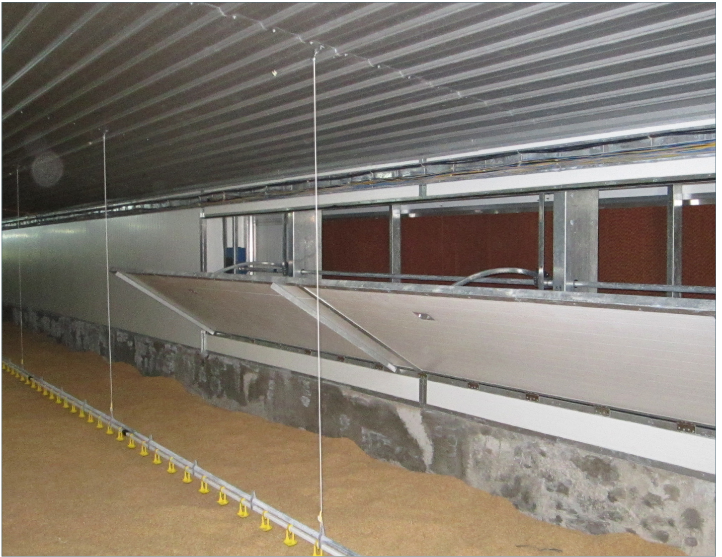
With a Rack & Pinion opening, a stable system is ensured with a solid closing mechanism.
